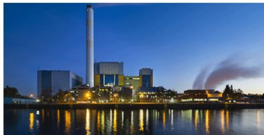
Flue Gas Cleaning
